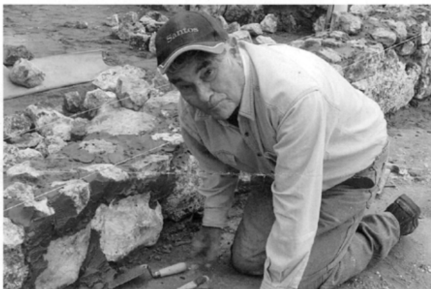
Malcolm Piggott hard at work building a stonewall.
