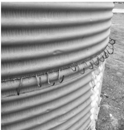
CUP HOOKS FOR THE SCHOOL STUDENTS STILL REMAIN ON THE RAINWATER TANK AT MOORLANDS HALL
