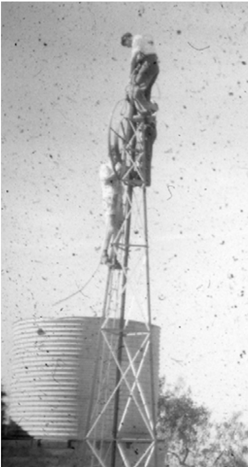
CONSTRUCTION OF THE LIGHT TOWER
